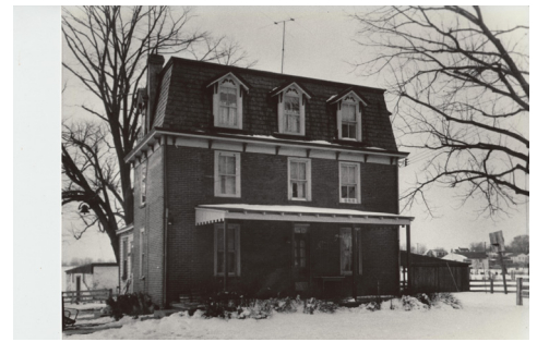
The former "Free Library of Aston" building (also former Sun Riding School)
